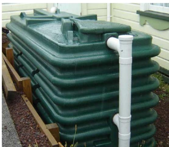
Rainwater reuse and detention tanks comprise two sections, above and below a small diameter orifice part way up the side of the tank. The volume below the orifice is used to store rainfall collected from roof areas for non-potable use within the building, while the volume above the orifice is used for detention and the orifice allows the slow-release of roof run-off during and after rainfall events.
